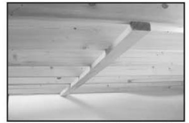
Mid-span nailer keeps joists straight, remove when project is complete.
